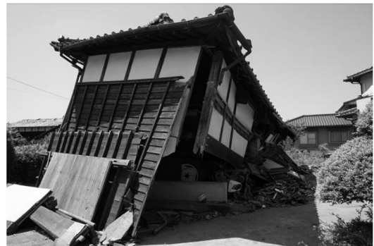
Fig.2. The damages of barns.
